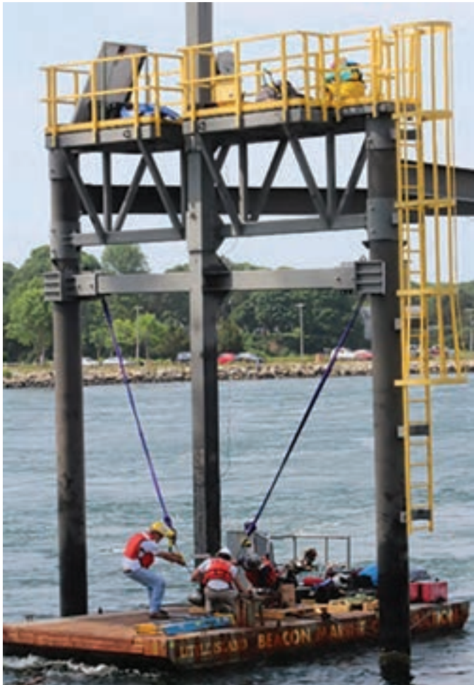
Rigging up to test a turbine at the Bourne Tidal Test Site in the Cape Cod Canal in Bourne, MA, USA.
