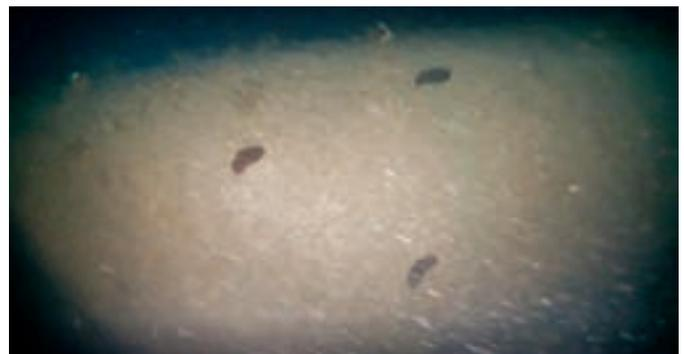
*Close view of the pipeline. In this image we could see biofouling on the pipeline. This is very common and does not present an issue. No cracks in the concrete casing were encountered.*
