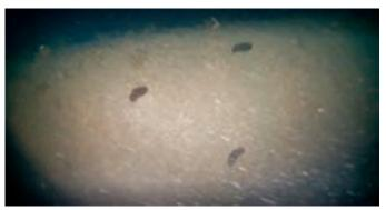
Close view of the pipeline. In this image we could see biofouling on the pipeline. This is very common and does not present an issue. No cracks in the concrete casing were encountered.
