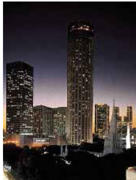
Fig.1 Raffles City Convention Centre and Swissotel-the-Stamford
