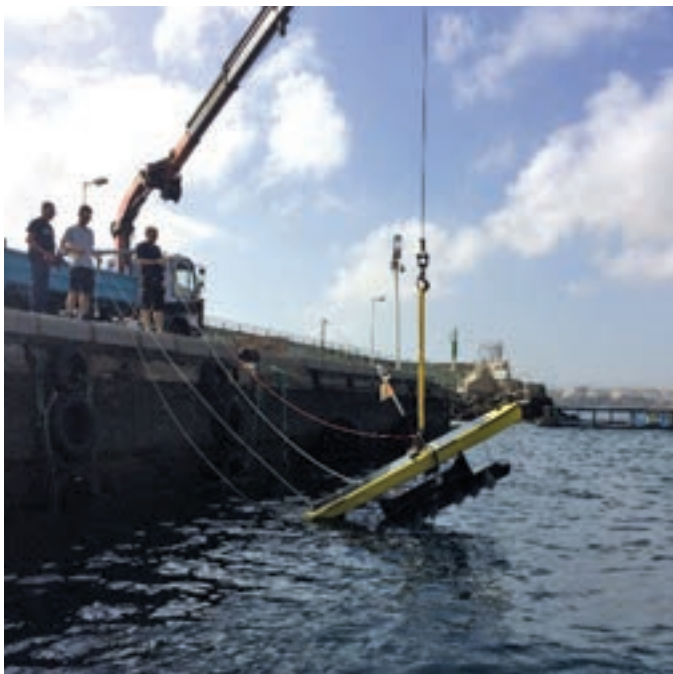
No vessel ever touched the Waveglider. The dockside crane handled launch and recovery.
